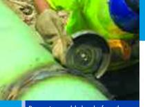
Removing weld slag before the next weld pass.
