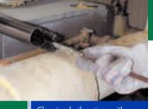
Cleaning boiler pipes with a flue brush.
