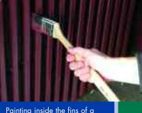
Painting inside the fins of a radiator with a Radiator brush.
